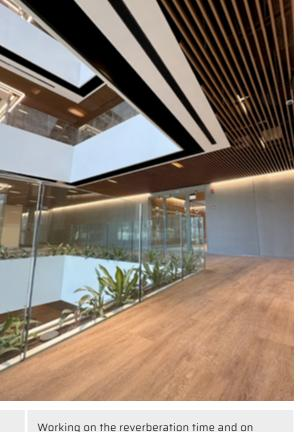
the intelligibility of speech, Metal Baffles with **perforated surfaces** and coupled with specific **sound-absorbing materials**, are an excellent technical solution to characterize the environment by improving the **acoustic** comfort. Customizable by finishing, colors and perforation mode, Metal Baffles are custom made systems, properly conceived to satisfy the specific requirements of each project.
